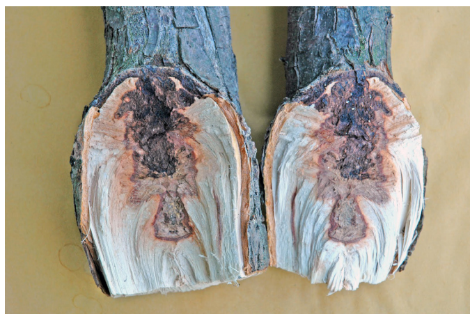
Cross-section of the same fork reveals bark trapped between limbs, preventing strong wood union and creating a weak point. Photo by William Reid
