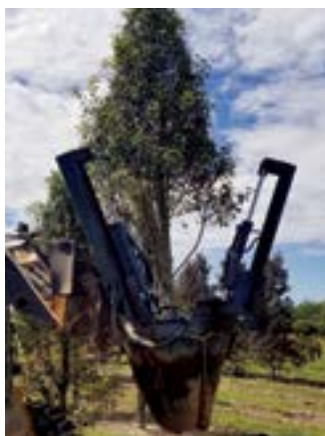
Trees and shrubs can be dug by hand or by using heavy machinery.
