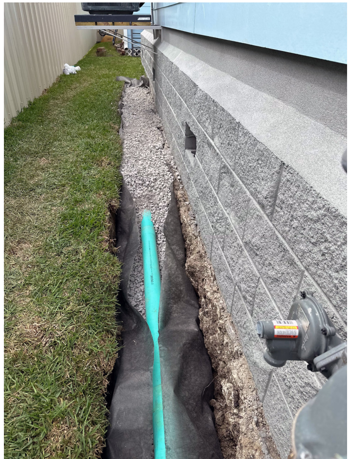
Installing perforated pipe and gravel.
