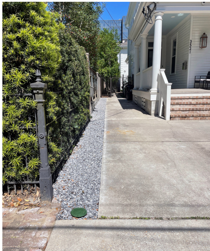
Drainage grates, at left, allow water to flow into the French drain, while pop-ups allow water to drain out downstream when pressure in the drain builds up.
