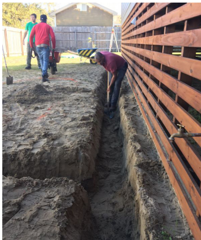
Excavating a trench for a French drain.
