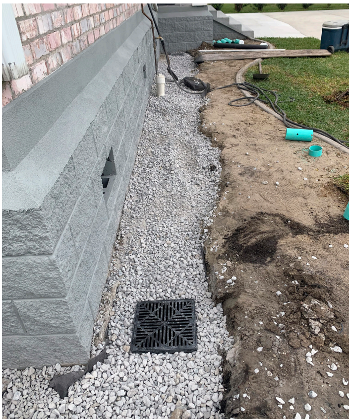
Drainage grates, at left, allow water to flow into the French drain, while pop-ups allow water to drain out downstream when pressure in the drain builds up.
