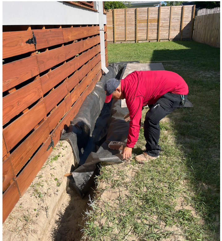
Lining a trench with geotextile fabric.
