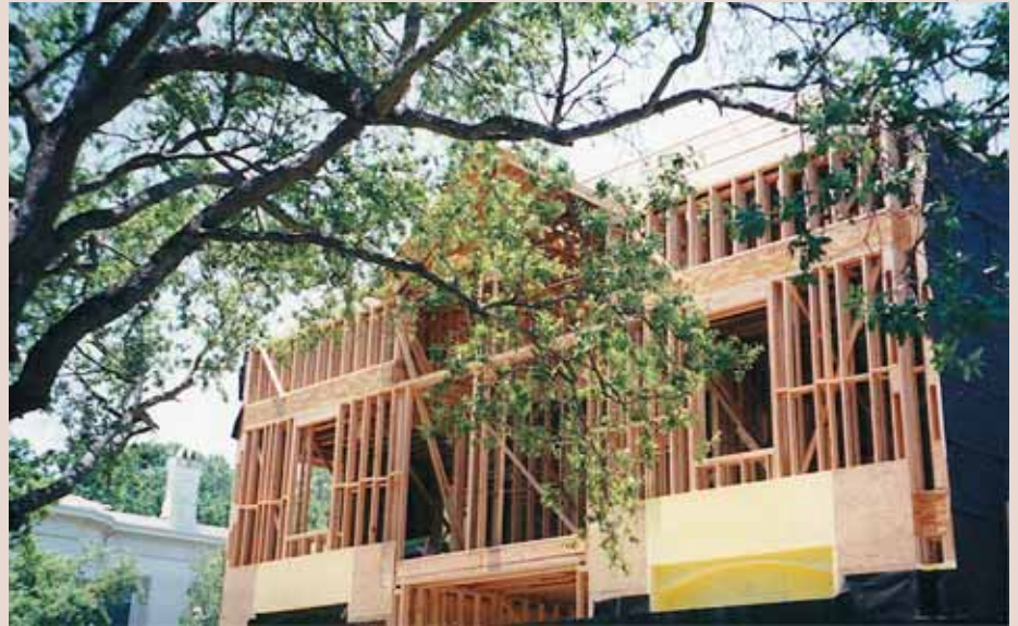
The Louisiana Forest Products Laboratory is testing wood treatments that will protect structural materials from termites. This house in New Orleans is being constructed with borate-treated lumber. Borates have been found to be toxic to termites.
