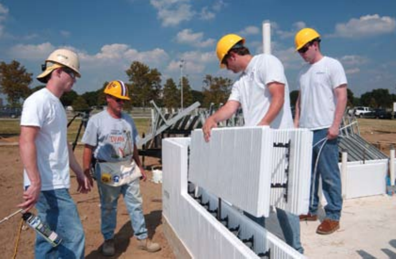
One building system features foam panels that can be locked together and filled with concrete to create strong walls with built-in insulation value.
