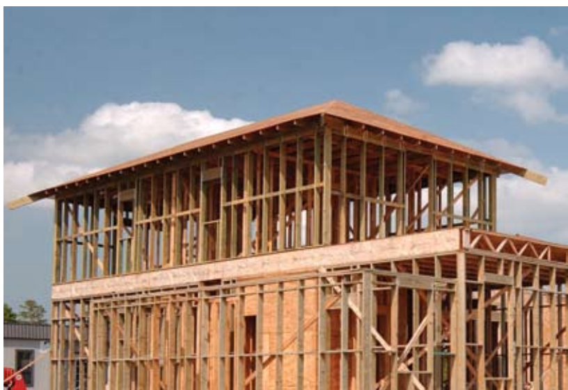
Stack framing using 2x6 wall studs placed 24 inches apart align with the rafters and floor joists to improve the process of tying the structure with hurricane straps, increase stability and increase energy efficiency.
