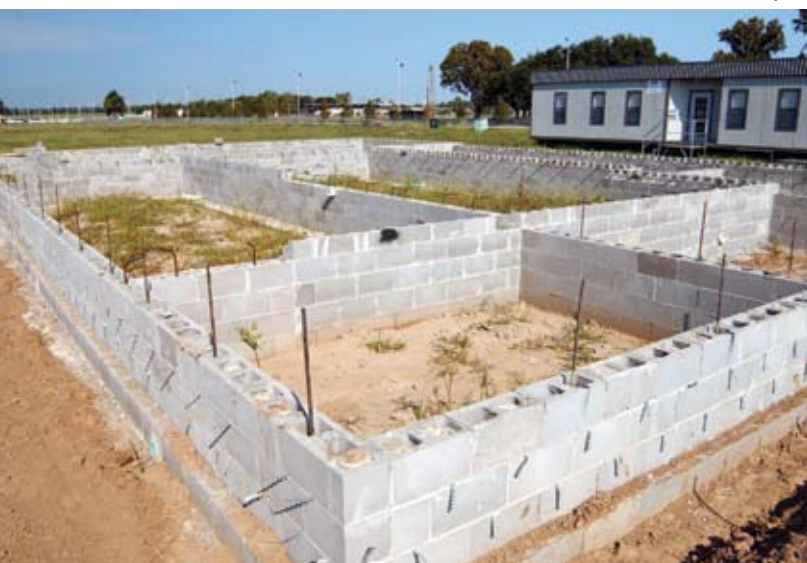
A rebar-reinforced concrete block stem wall is filled with compacted soil and covered with a concrete slab cap to comprise one of the elevated foundation models.
