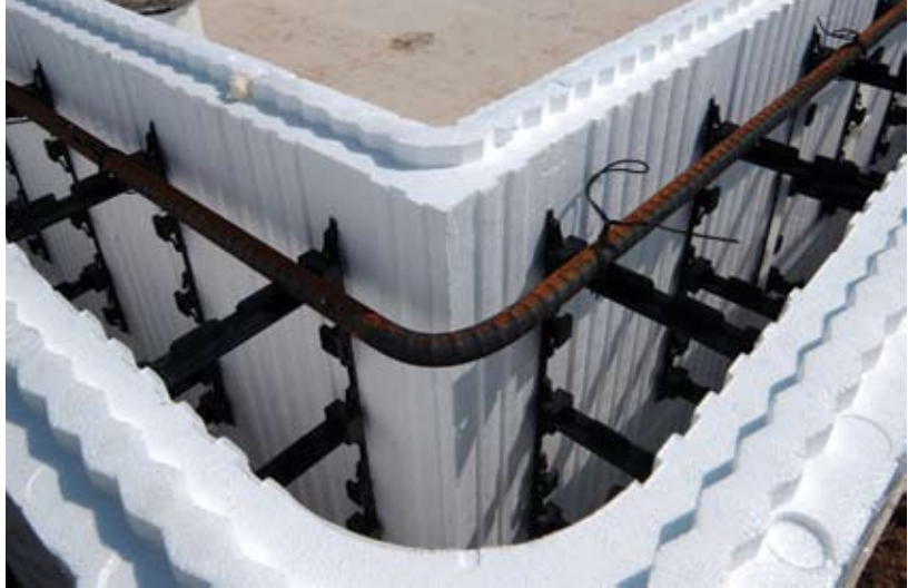
The insulating concrete forms (ICF) are held together with reinforcing steel bars, which add strength to the walls when the concrete is poured.
