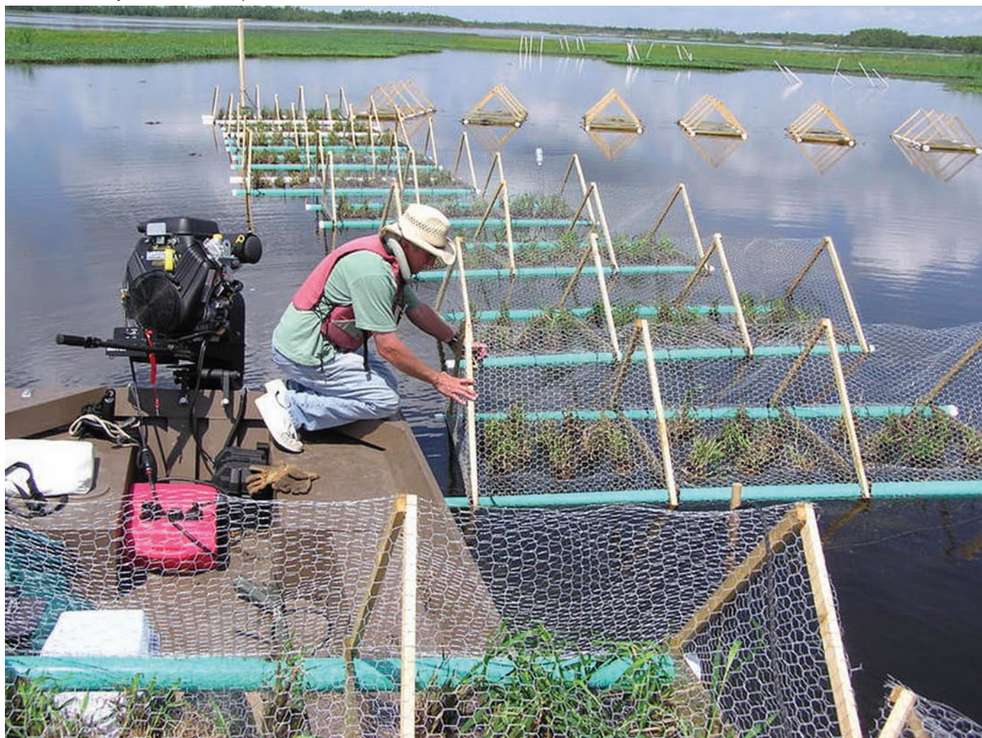
Figure 5. Deployment of vegetated artificial floating marsh system structures at the Mandalay marsh site in April 2006.
