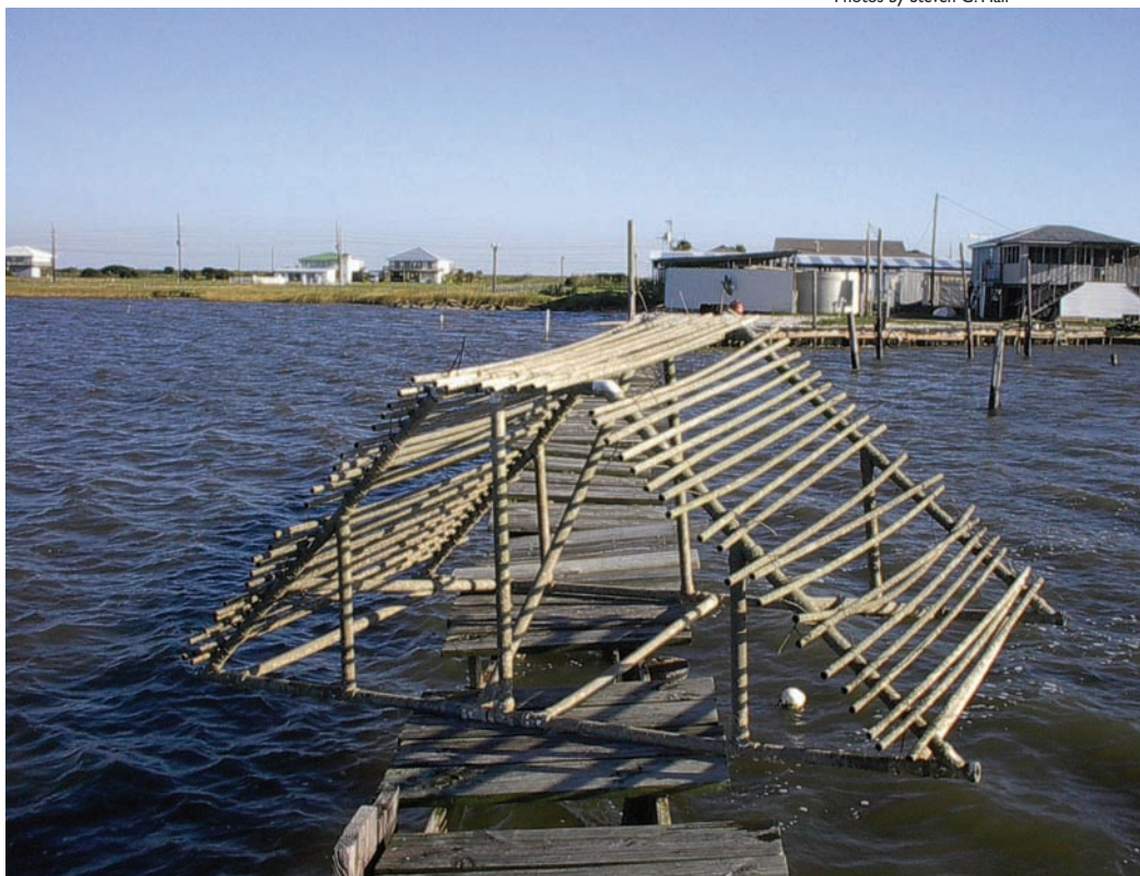
A section of a full-size oysterbreak (above) was built and deployed at the LSU oyster hatchery facility at Grand Isle in 2004. The structure is made of "French tube" – expanded and corrugated PVC. The 5-foot-high structure was placed in the water (below) to evaluate its ability as a home for oysters. The area behind the oysterbreak contains a "long-line" system that allows oyster producers to pull up and lower down materials on which oysters live. The area where the oysterbreak was tested allows the structure to be slightly submerged at low tide.
