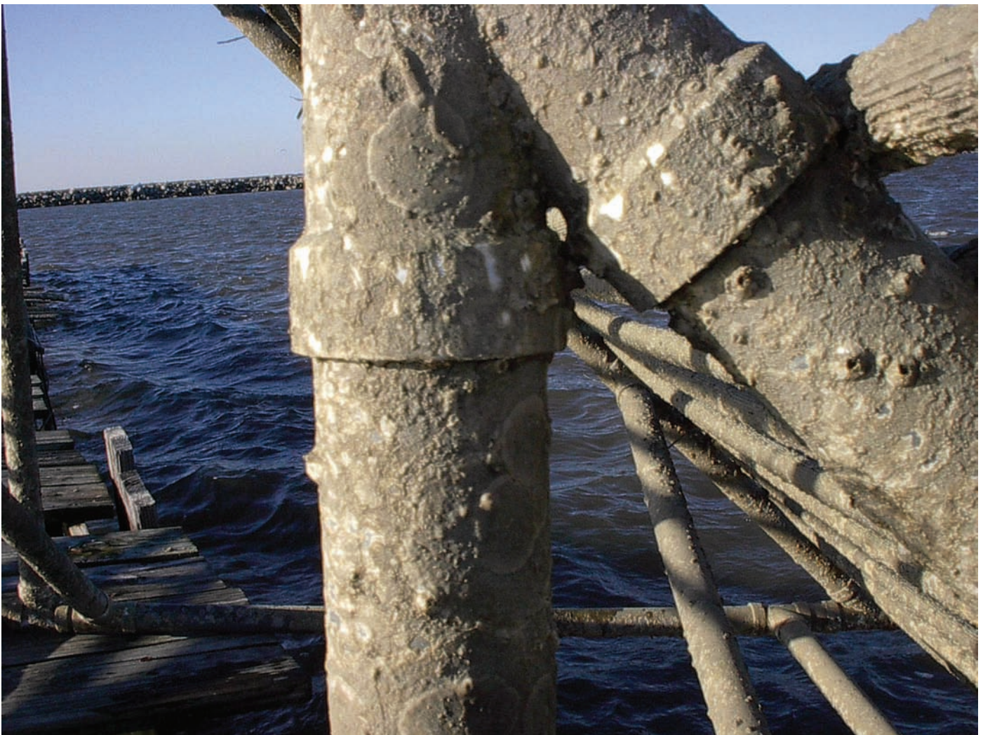
An early oysterbreak was made of "French tube," expanded and corrugated PVC pipe (above). The material provided habitat for oysters and barnacles as seen in the photo below. Other materials, however, have proved to provide a better place for oysters to live.
