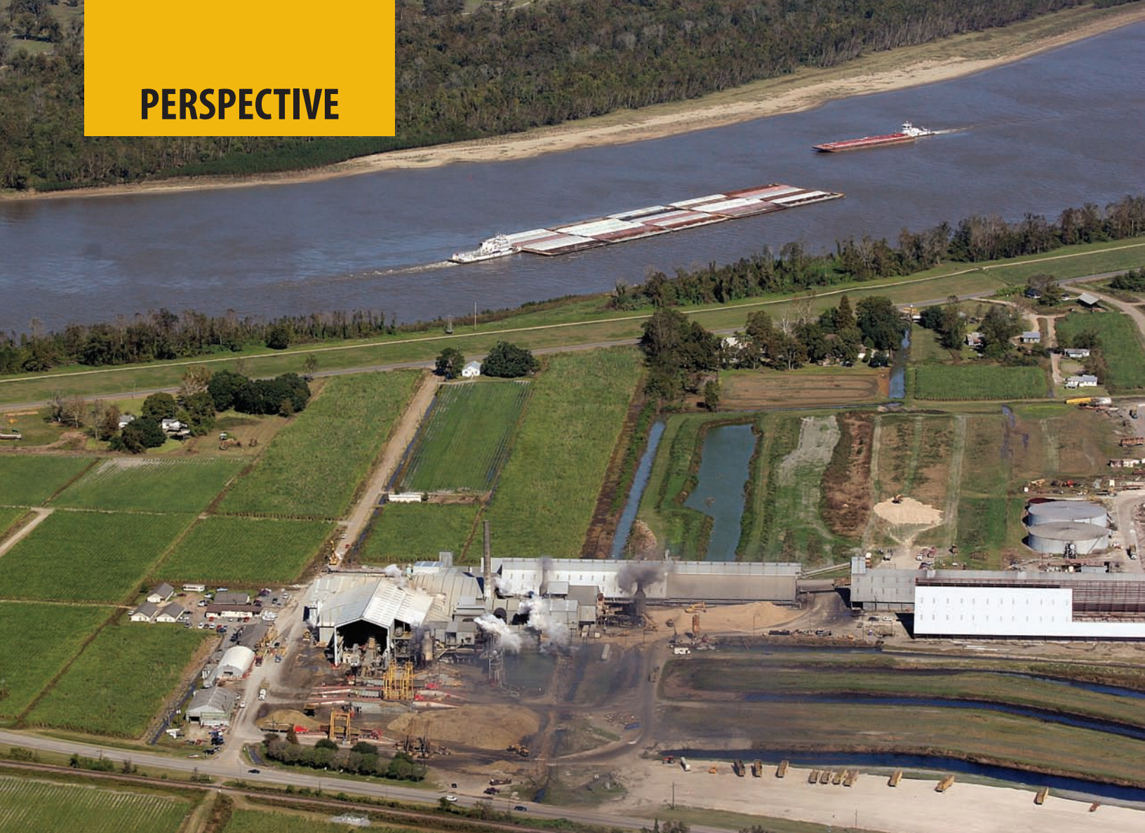
The Cora Texas Manufacturing Co. sugar factory at White Castle, La., is near the Mississippi River.
