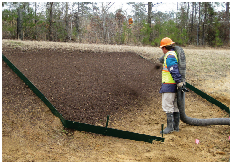
Compost/mulch application to test plots along I-49 via blower truck in Rapides Parish. Photo by David C. Weindorf
