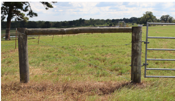
Wooden H-brace. Photo by Abby Dunn
