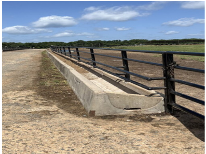
Permanent feedlot feed bunk. Photo by Tripp Morgan
