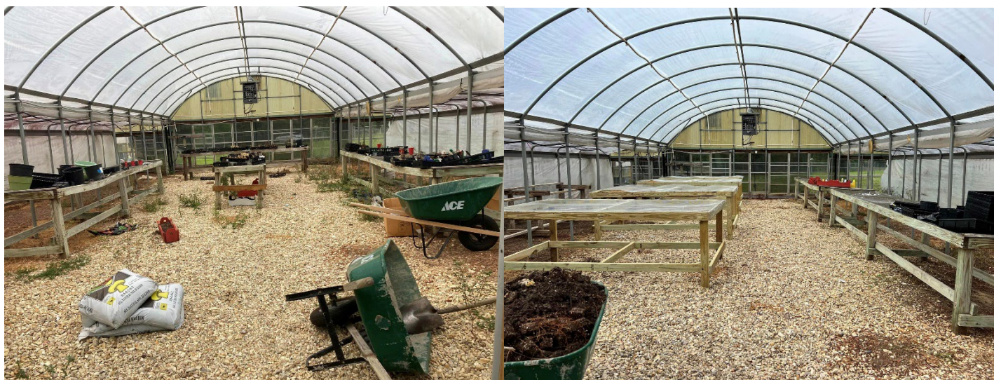
Before and after cleanup of Doyle High School greenhouse and installation of new greenhouse benches.
