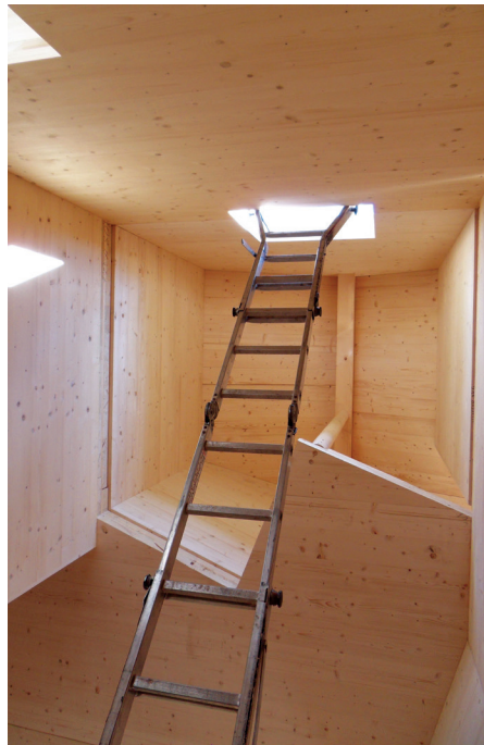
Cross-laminated timber construction.
