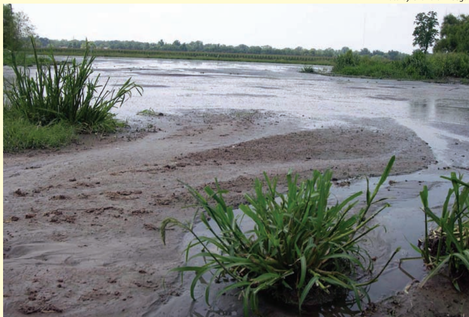
Figure 1. Bedding sand and dairy manure fill up an anaerobic lagoon, seriously undermining the bacterial treatment process. Land-applying the untreated water or waste on adjacent land leads to excess nutrients and bacterial contamination in nearby water bodies.
