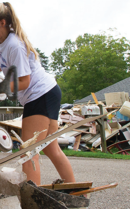
In the aftermath of the August 2016 flood that struck south Louisiana, 4-H'ers helped gut damaged houses. Cameron Parish 4-H'ers Kailey Murrell, left, and Hannah Doucet dump a wagon full of discarded drywall and insulation, adding to an ever-growing pile of flood-damaged items outside the Denham Springs, Louisiana, home they helped clean. Photo by Olivia McClure
