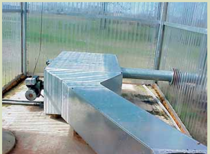
Figure 2. One modification is to use a floor heater connected to an 18-inch duct for heat transfer.
