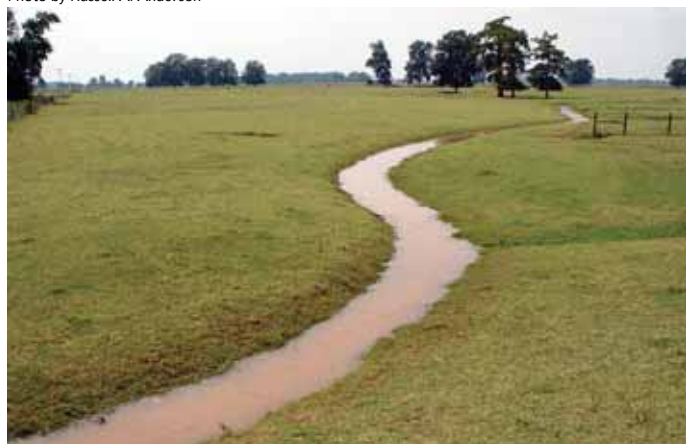
This is one of the drainage ditches carrying runoff from the 400 acres of agricultural production at the Red River Research Station to the constructed wetland between the fields and the Flat River.
