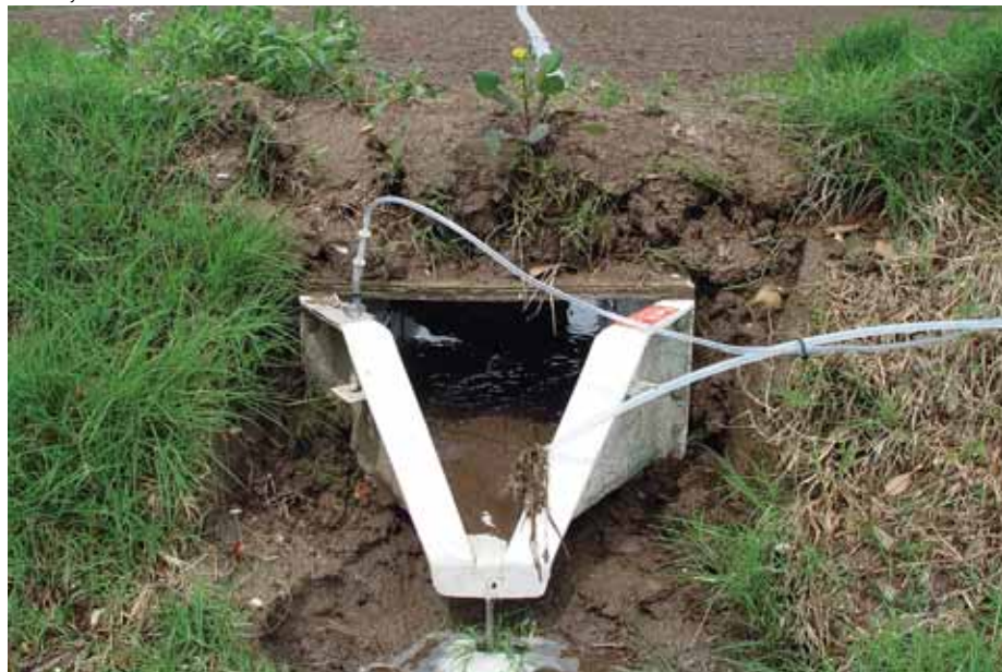
This is called an H flume. They are installed in the levees and used in the project to collect runoff. Note the tubing that runs to the collection container.
