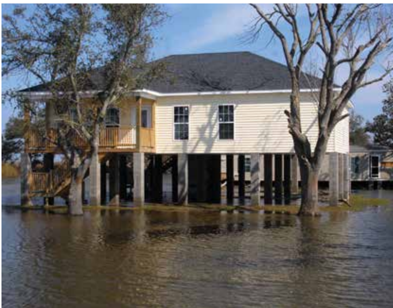
A raised home in Cameron Parish was undamaged by the floodwaters of Hurricane Ike in 2008. Photo by Bruce Schultz
