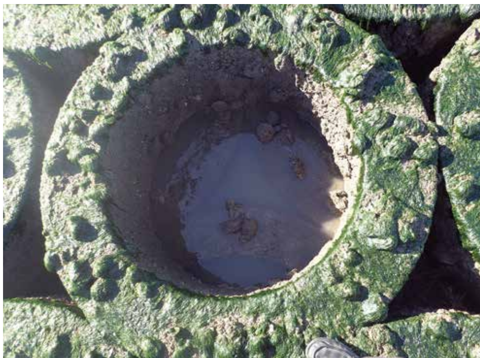
The rings are 5 feet in diameter with 9-inch walls and provide habitat for barnacles, oysters and algae, while encouraging the settlement of sediment behind and below the structure. Photo by Steven G. Hall
