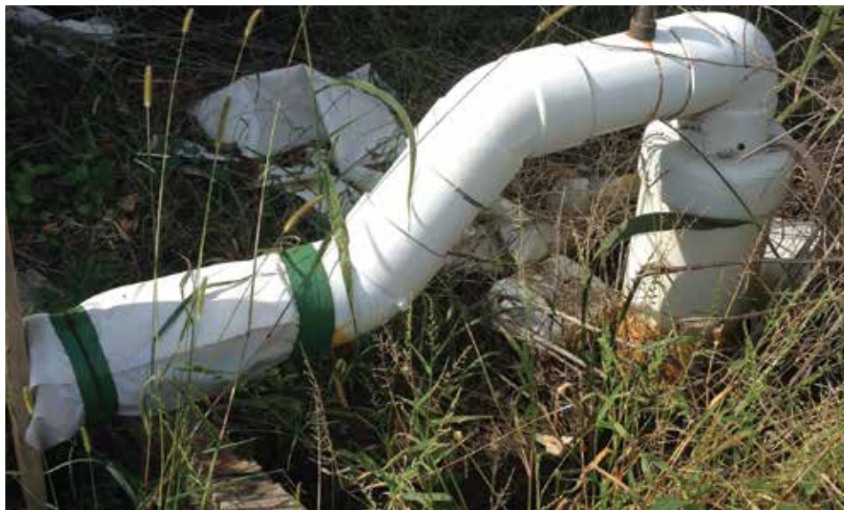
This is an example of a poorly maintained well. The area surrounding a private well must be free of contaminants. Photo by Achyut Adhikari
