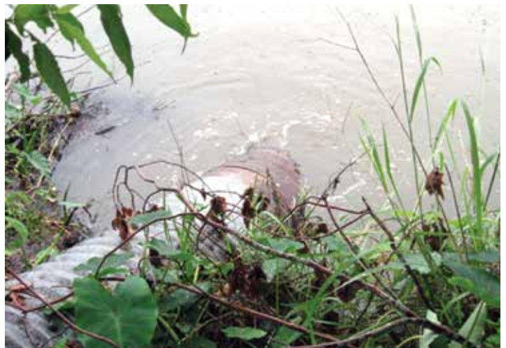
Figure 2. Stormwater drains around University Lake carry sediments, nutrients and other chemicals into the water body. Photos by Y. Jun Xu
