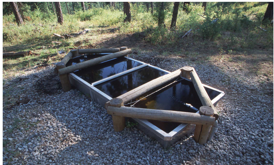
Soil stabilization is critical around water troughs.
