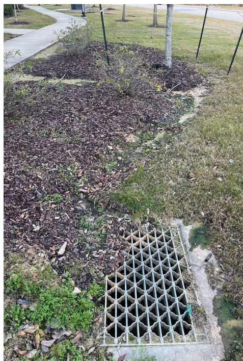
Beds without landscape edging may have mulch washout in the rain, potentially causing downstream clogging.
