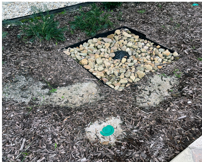
Edging can keep different materials separated, which maintains the material aesthetic and may be useful in protecting drainage features from clogging.
