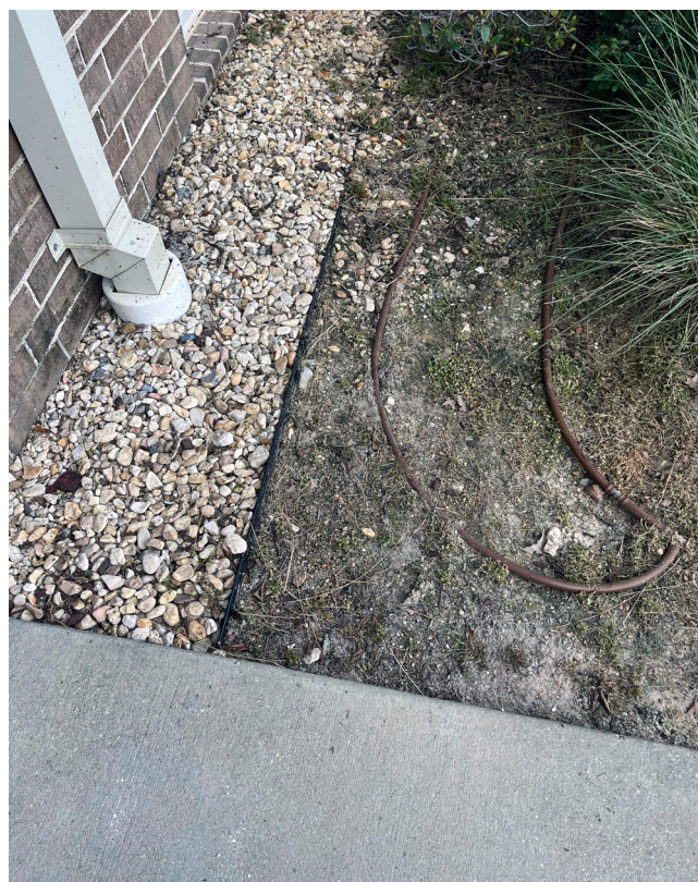
Plastic edging is an affordable alternative for low traffic areas to keep materials separated.
