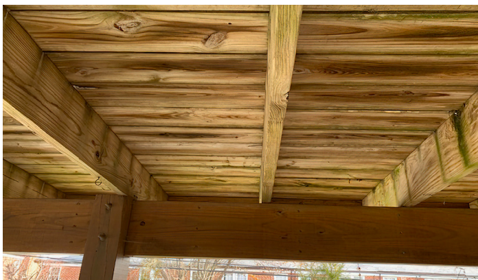
Image 1: Underside of a deck. Photo by Gretchen Gerber.
