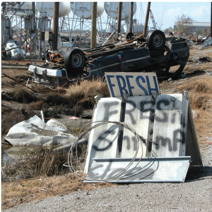
Damage in Cameron Parish after Hurricane Rita hit the coast in 2005. Photo by Kevin Savoie
