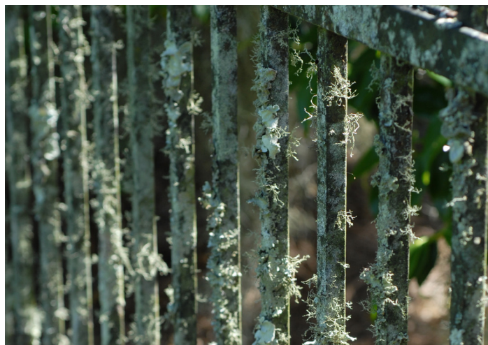
Lichens growing on an iron fence post.
